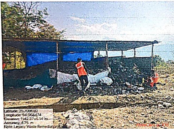
Sorted Waste stored for further disposal: Ongoing
